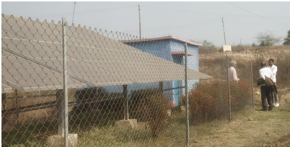
Figure 4: Solar Lift Irrigation Infrastructure-Rajhara Kothi
